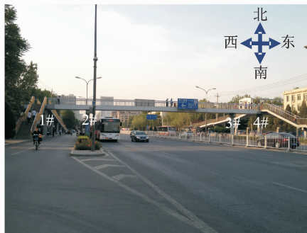
图 4 北京工业大学西门人行天桥 Fig. 4 Footbridge at the west gate of Beijing University of Technology
