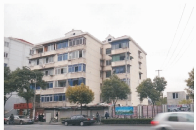
(b) 6层居民建筑北视图 (b) North view of six-story residential
