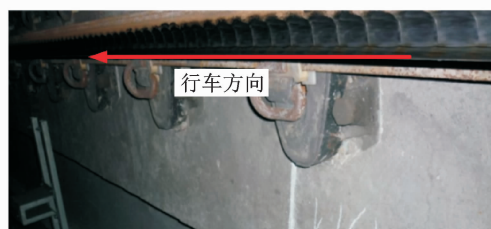
(a) 钢轨波磨区域 (a) Rail corrugation area
