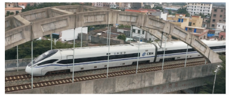
(a) 现场行车试验 (a) Field traffic test
