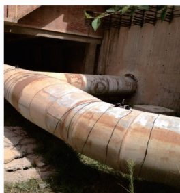
(a) 现场测点布置图 (a) Field test of pipeline
