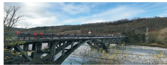
(a) Lamberti拱桥全貌图 (a) The overview of Lamberti arch bridge
