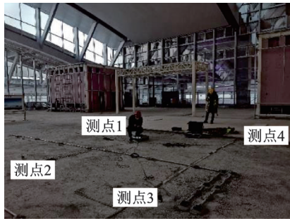
(a) 高架候车厅 (a) Elevated waiting hall
