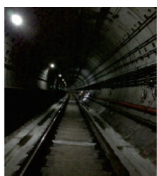
(a) 监测现场 (a) In-site monitoring
