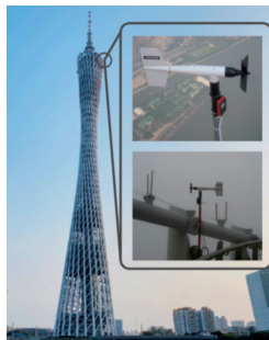
图 10 广州塔风速传感器布置 Fig.10 Wind speed sensor layout of Canton Tower
