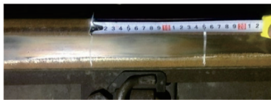
图3 A-B区间线路情况 Fig.3 Line condition of A-B section
